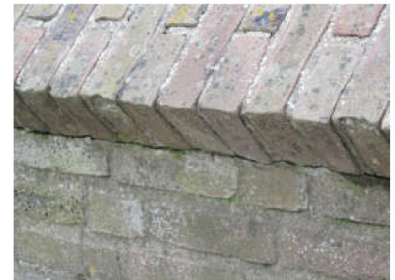
Rollaag - losgescheurd
