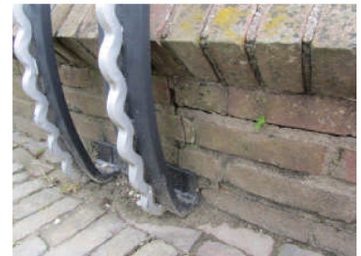
Rollaag - losgescheurd
